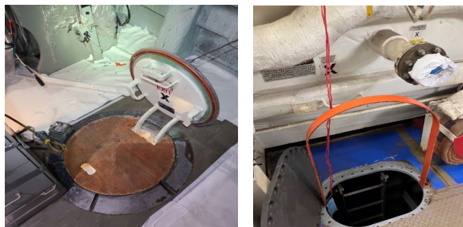
(Left) Image shows a hatch cover with adequate covering. (Right) Image shows appropriate use of a "U" bar to temporarily guard flush manholes during shipbuilding and ship repair operations.
