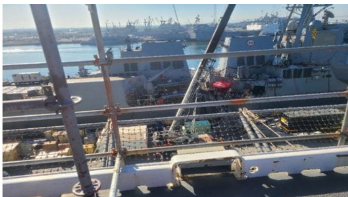
Image shows use of a guardrail at the deck's edge to prevent workers from falling to a lower level.
